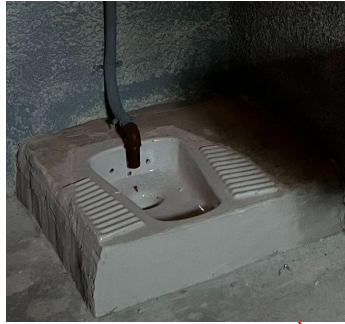
Squat toilet (non-functional)
